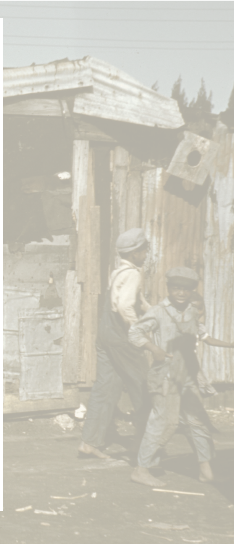
Housing of Black migrant workers. Florida. (1941)
